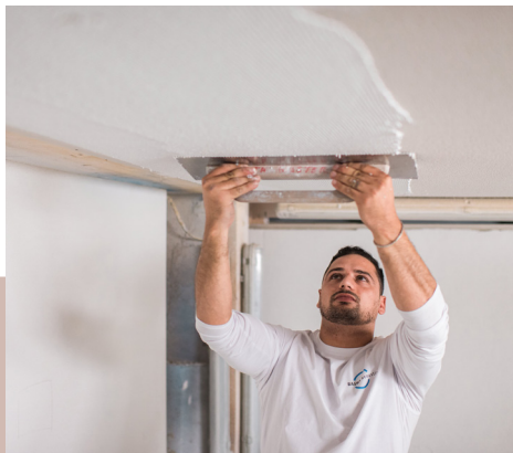
BASWA System Installation
